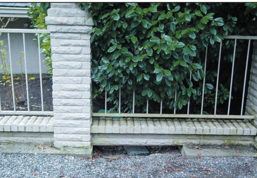
Meter is located underneath the fence. The fence or the meter needs to be relocated.
