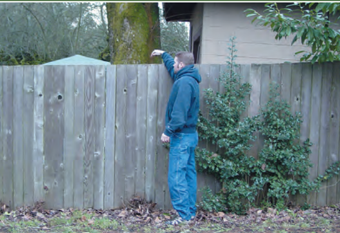
Meter is located behind the fence. The fence or the meter needs to be relocated.
