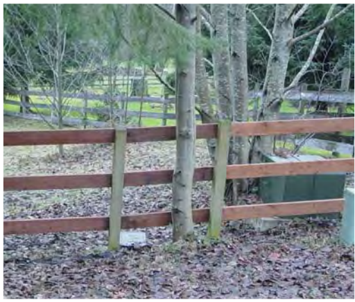
Meter access is obstructed – it's located inside the fence
