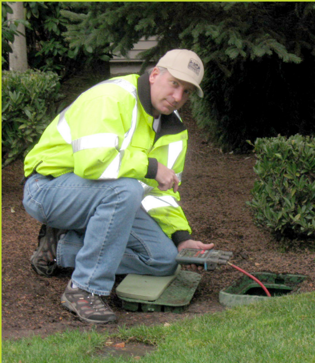
A Backflow Assembly Tester will test and certify your backflow assembly for you.
